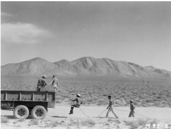
Laying cable for Uncle
